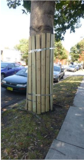
Example image of acceptable tree protection batters
